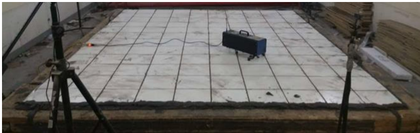
Photo 1: View of Source Chamber, finish flooring installation observed
