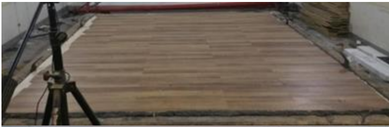
Photo 1: View of Source Chamber, finish flooring installation observed
