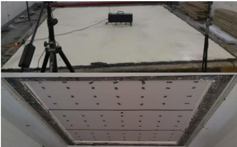
Photo 1: View of Source Chamber, finish flooring installation observed
