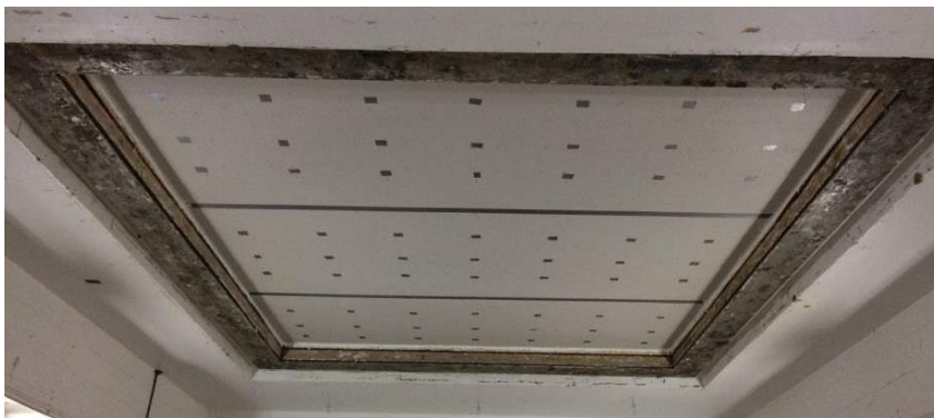
Photo 2: View of Receive Chamber
