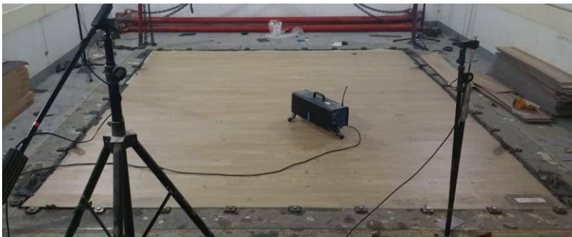
Photo 1: View of Source Chamber, finish flooring installation observed
