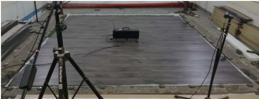
Photo 1: View of Source Chamber, finish flooring installation observed
