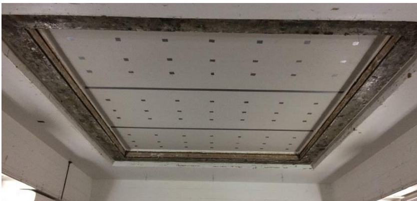
Photo 2: View of Receive Chamber
