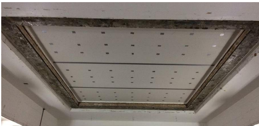
Photo 2: View of Receive Chamber
