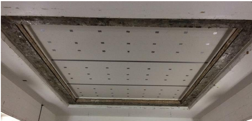
Photo 2: View of Receive Chamber
